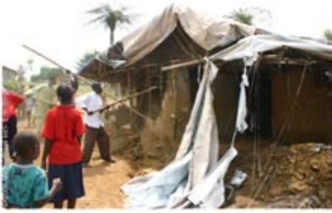
destroying the old structure...
